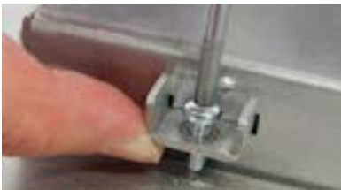
Figure 12: Fastening the Clamping Bracket
